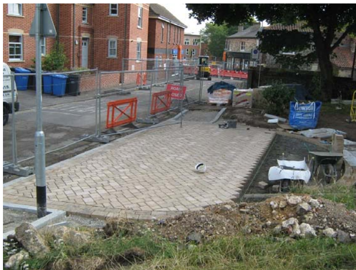
Construction of turning area on Bakers Road
