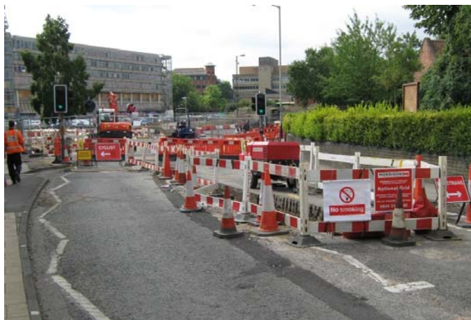
Gas main replacement at southern end of St Augustine's Street
